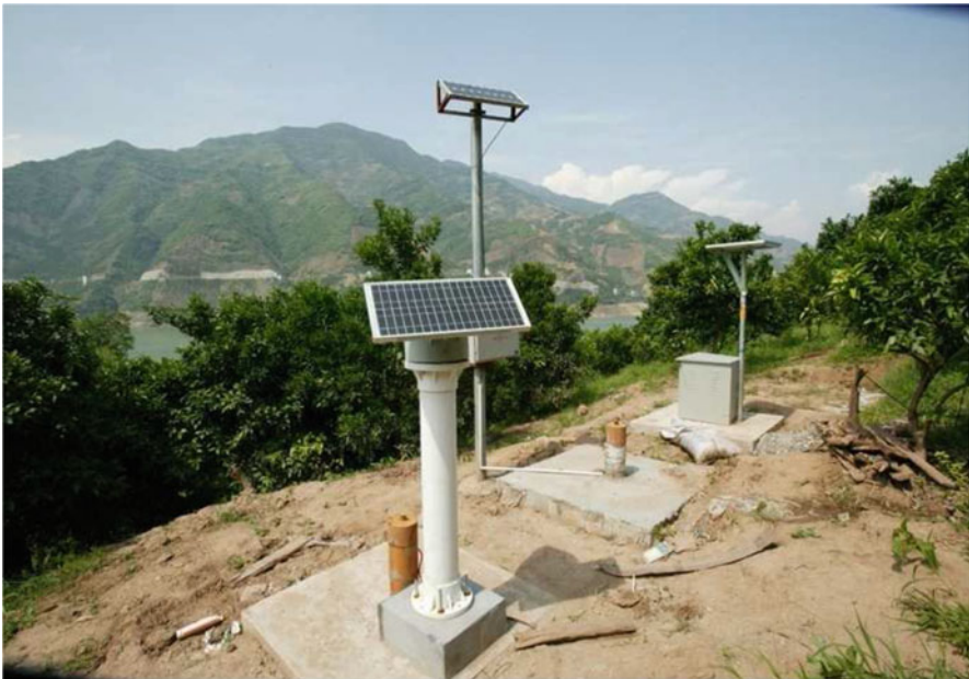
Fig. 3.6 Detecting landslide thrust and groundwater level
